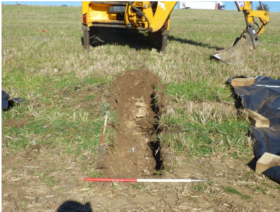
Soakaway 28, general view, looking north
